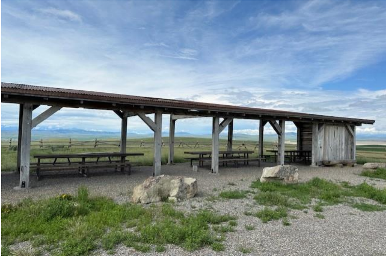
Figure 27: Recreation Infrastructure at Copper City Trailhead - Butte FO 2023
