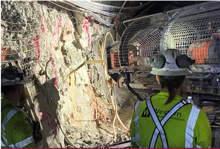
Underground drilling operations in the Sunday Mine Complex.
